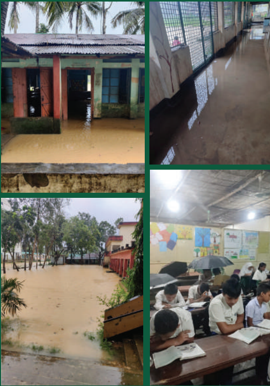
Photo: Floodwaters submerge the school playground and ground floors; students attend classes under umbrellas, as rain seeps through the roofs.
